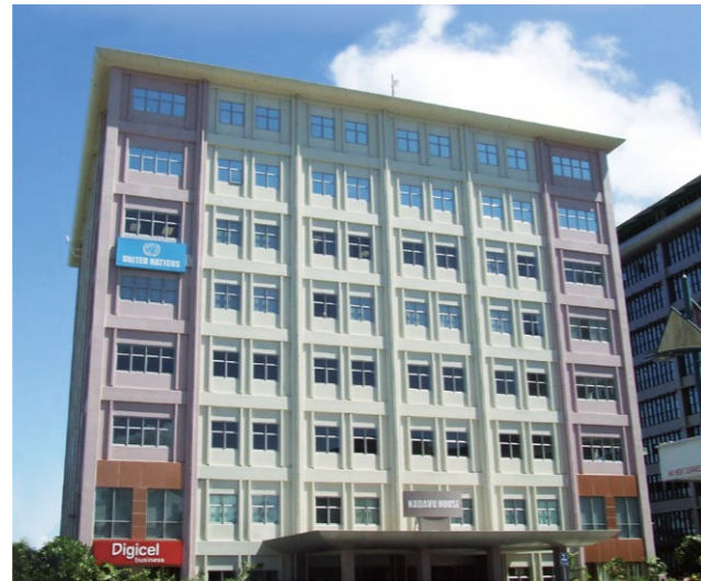
Kadavu House United Nations Office, Suva, Fiji
