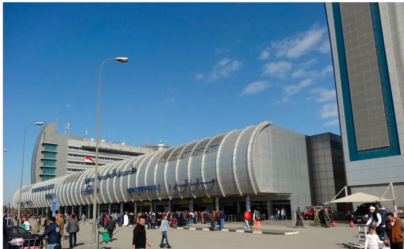
Airport international T1,Cairo,Egypt
