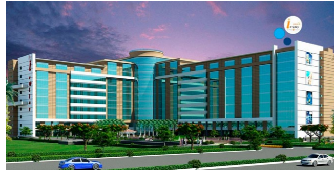
I-Valley technology building, India
