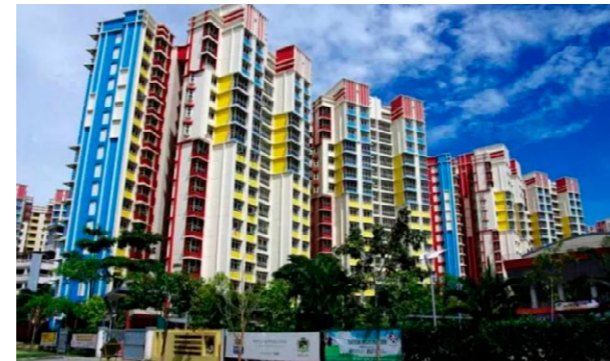
HDB 27th Tender Lift Project, Singapore
