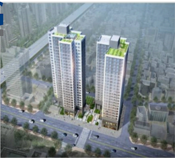
Jegi-dong Station Complex...
